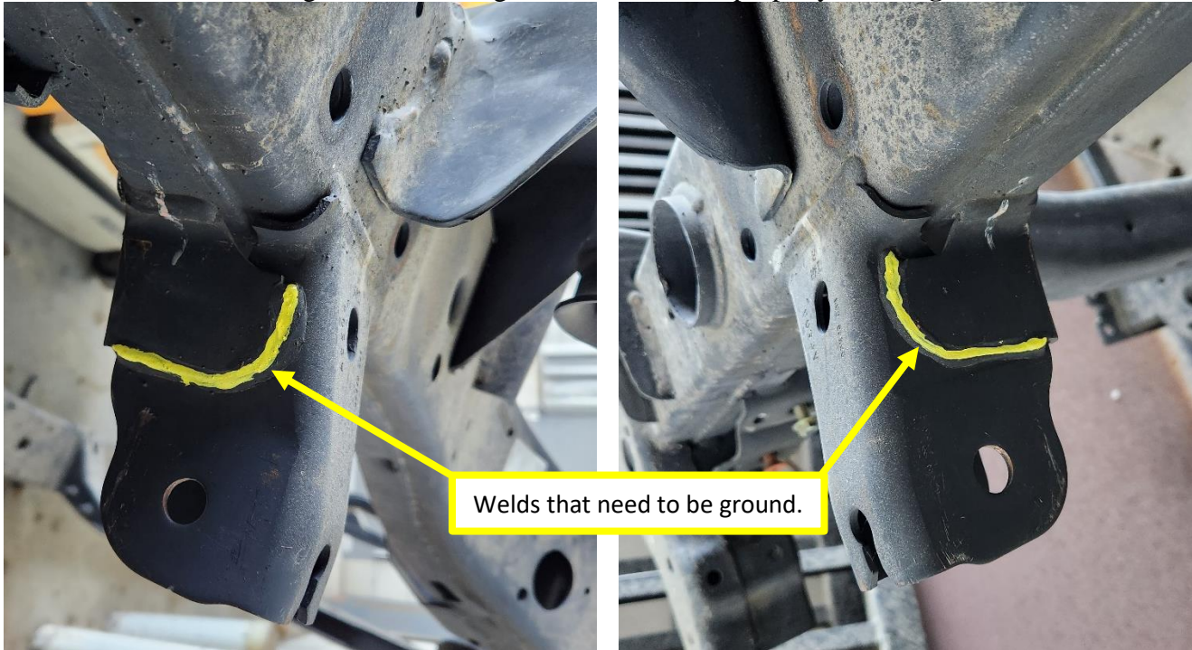
Figure 7. and 8. Track Bar Bracket Welds That May Need to be Ground Down
