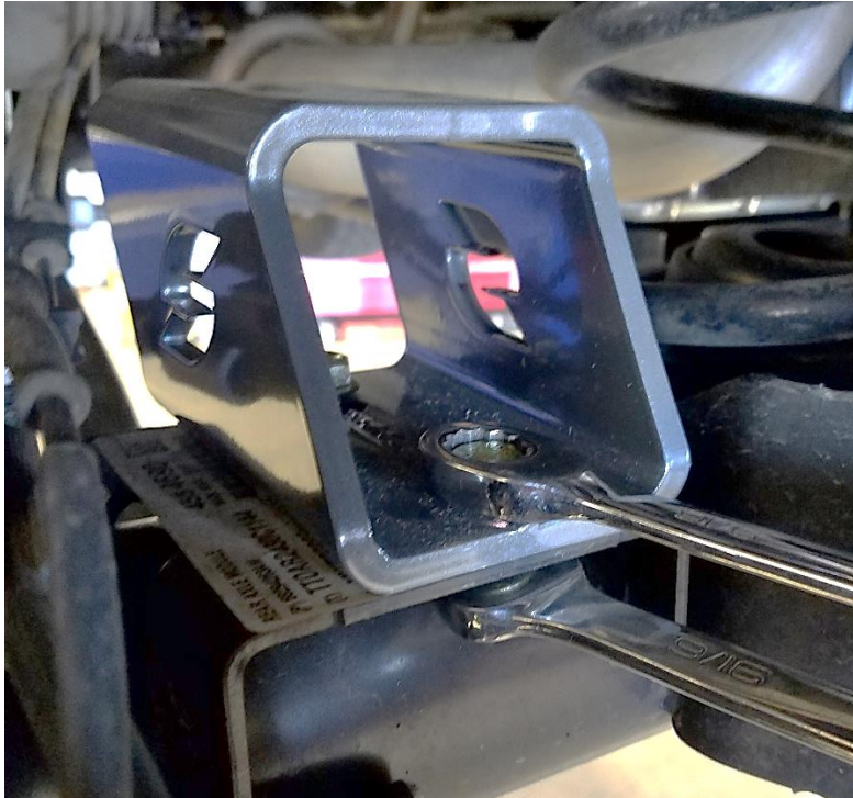
Figure 2. Tightening the Bumpstop Extension Bolts.
