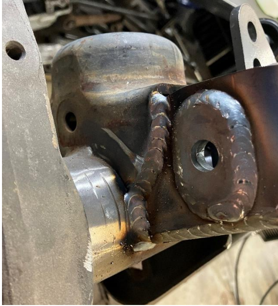
Figure 7. Vertical Weld on the Spring Perch
