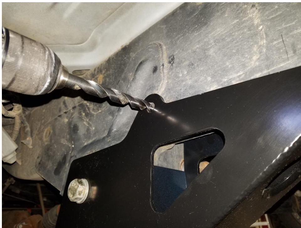
Figure 6. Using a Drill to Mark Hole Locations
