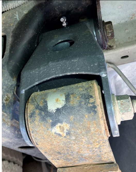
Figure 5. Upper and Lower Shackle Assembly Bolt Installed.
